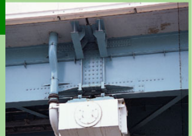
Connecting bridge girders
