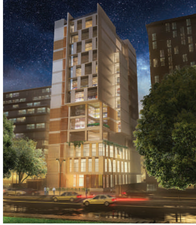
ONGOING Commercial Complex SIZE: (250-2577) sft.
