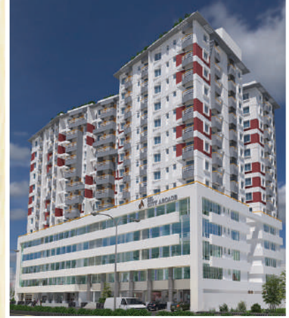
ONGOING Commercial cum Residential Complex SIZE: (252-2093) sft.
