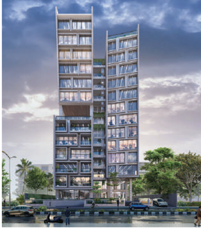
ONGOING Commercial Complex SIZE: (2248-3339) sft.
