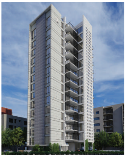
ONGOING Commercial Complex SIZE: (2248-3339) sft.
